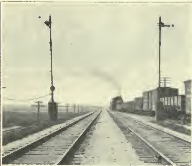
FIG. 285. SIGNALS. Double track automatic signals on the Chicago, Milwaukee & St. Paul Railway, near Healy Station.
